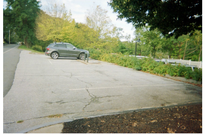
Bella Point Upper Parking Lot
